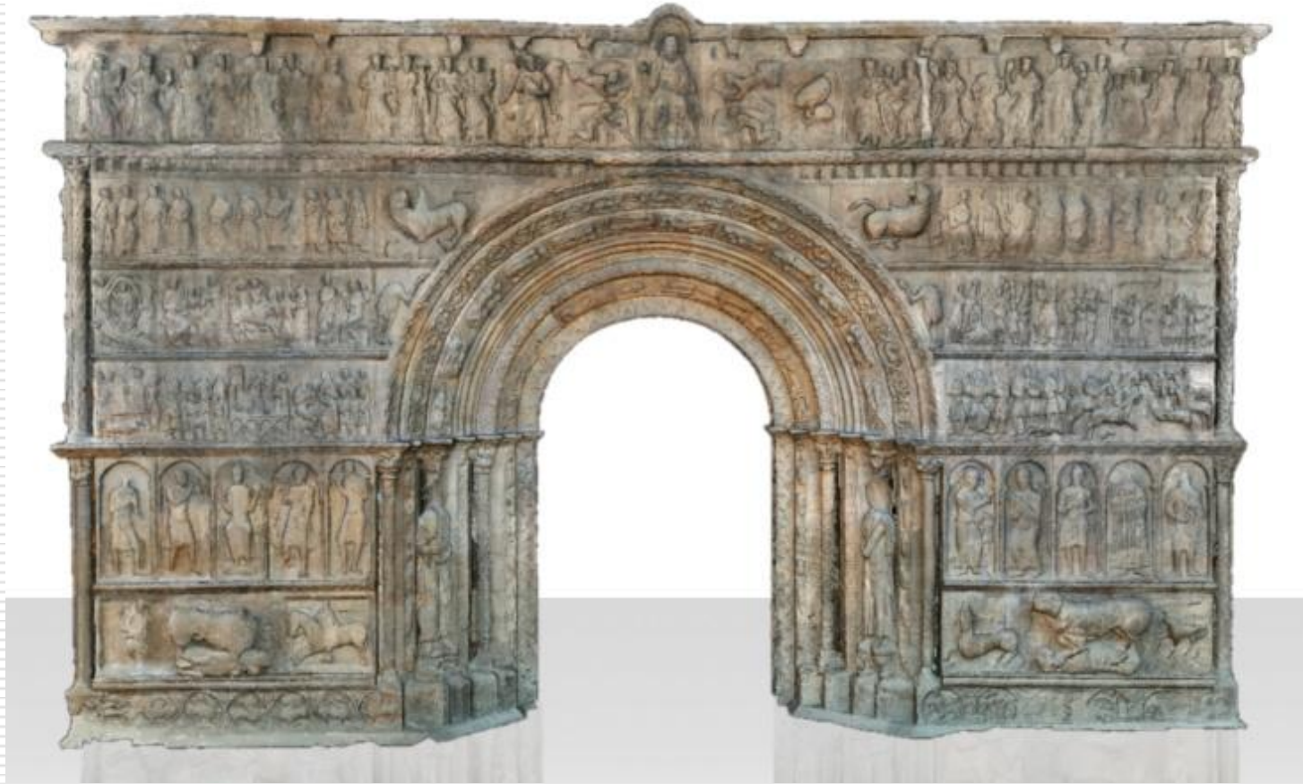
Portalada, monastery of Santa Maria De Ripoll, Spain 7 x 11 meters... to be scanned at 1mm resolution
