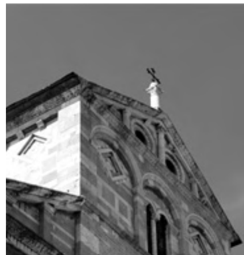
Fig. 1.7 Capital (replacement) with Pisan cross. Pisa, Duomo, end of the north transept
